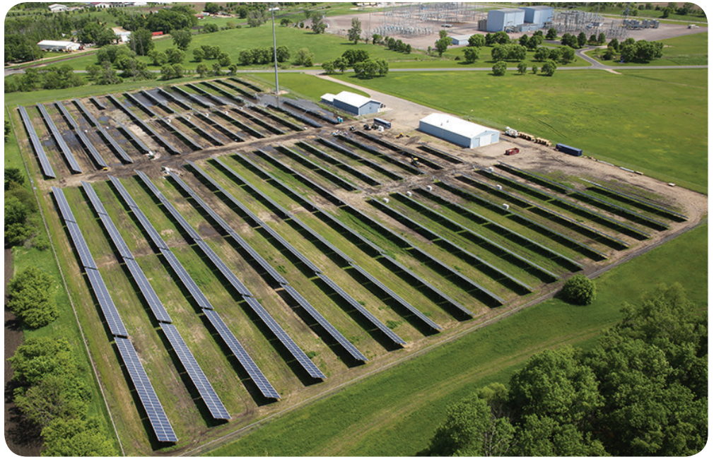
The Dickinson Solar Project (above) south of Buffalo was energized earlier this month. The 8,360 panels that make up this array are expected to add 2.25 megawatts of solar electricity to Wright-Hennepin's energy mix.
