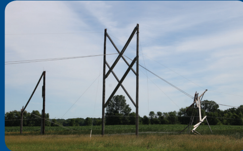
The photos above were taken near our Trail Haven substation. Xcel Energy's lines fell on WH's, leaving many in the area without power.
