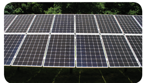
Wright-Hennepin's third solar community is mounted on the north side of the cooperative's campus in Rockford, Minn. This project was energized earlier this month, and consists of approximately 500 panels that produce 225,000 kWh to members who subscribe to the program.
