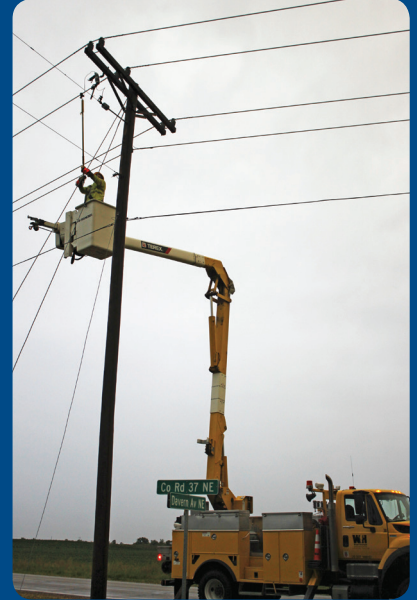
WH crews worked round-the-clock to repair damaged poles and lines, and restored power to all members by July 7.
