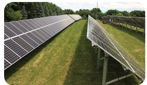
The Dickinson Solar Project (above) south of Buffalo was energized earlier this month. The 8,360 panels that make up this array are expected to add 2.25 megawatts of solar electricity to Wright-Hennepin's energy mix.
