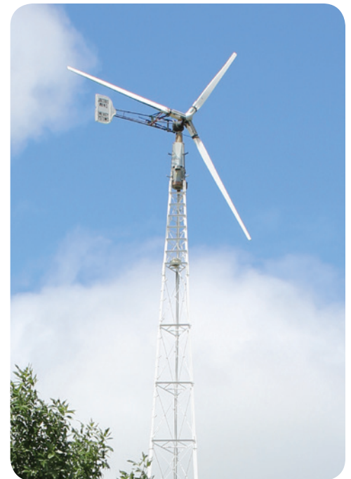
The wind turbine located on WH's campus will be dismantled this month.
