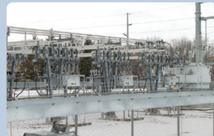
Wright-Hennepin will double the size of its Plymouth substation in 2017 to address rising energy needs.
