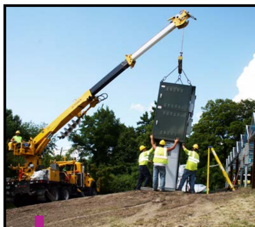
WH linemen assembling a battery cabinet.
