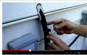
Stopping air infiltration from the outside
