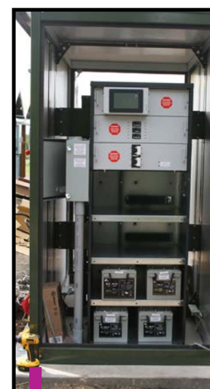
View of a battery cabinet filled with Silent Power storage units.
