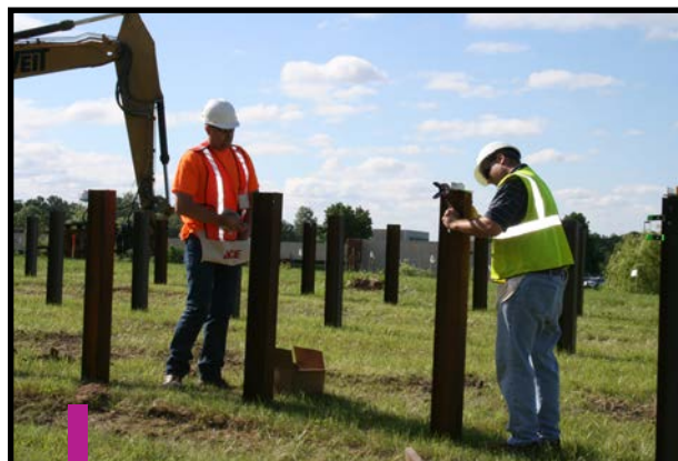
Construction workers drilling steel columns into the ground for the WH Solar Community array.
