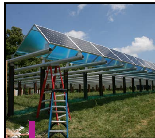
Front row of solar panels as they were being constructed on the WH Solar Community.
