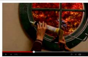
Caulking to reduce air leaks
