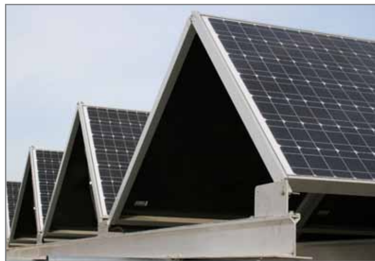
tenKsolar's design includes strategically placed reflector panels that allow the solar panels to increase their total energy production by 50 percent.
