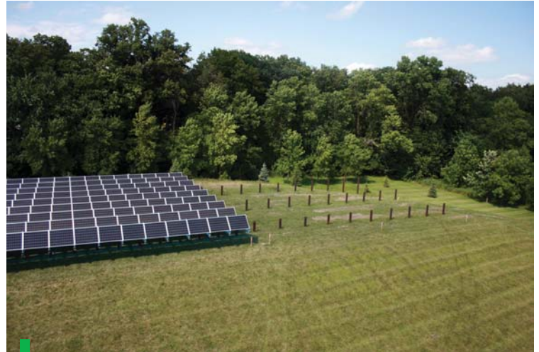
The groundwork for the second WH Solar Community was completed during the construction of the first community.
