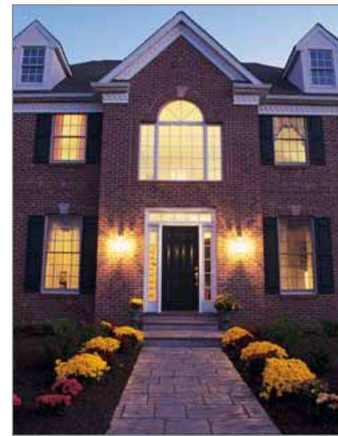
Make sure shrubs are trimmed back near your doors and windows so that burglars won't be able to hide behind them.
