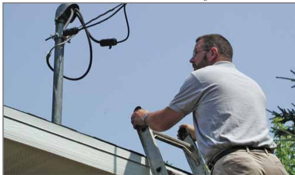
Be careful when working with ladders and scaffolding, making sure that these tools do not come into contact with power lines.
