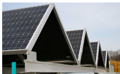
View of the TenKsolar panel system which consists of solar panels and reflectors. This is the system that will be used in the WH Solar Community array.
