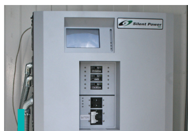
Front view of the Silent Power battery storage system. These batteries will be used to store the excess solar energy during the day.
