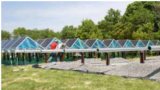
WH is in the process of constructing a second solar array located next to the first solar community project.
