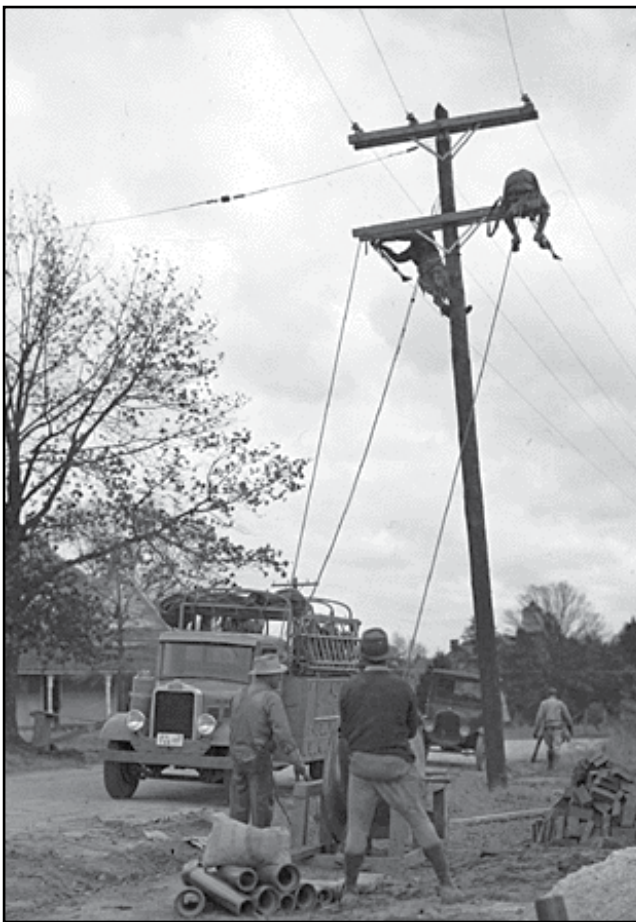
Line crews are shown working on a distribution line in the early days of the cooperative.
