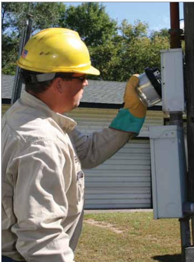
The metering department works to keep the smart-meter system functioning properly at all times to ensure accurate, timely meter reads.
