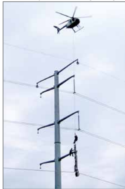
As a part of the stringing process for the CapX2020 project, line workers were transported from pole to pole via helicopter.
