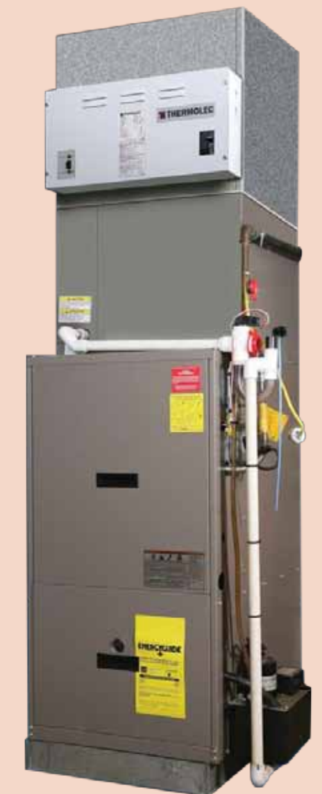
Plenum heaters can be easily added to an existing heating system and allow you to switch from your current fuel source to electric heat. The white device in the above photo is the actual unit, which is installed in the duct work of a furnace system.
