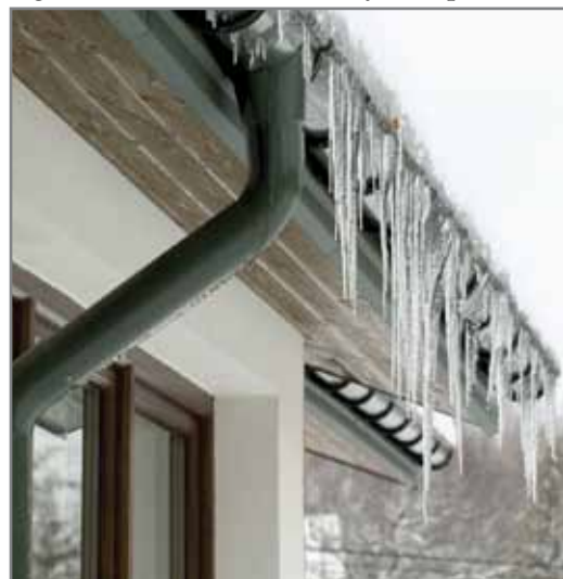
A roof melt system will help prevent ice dams and icicles from damaging your roof.
