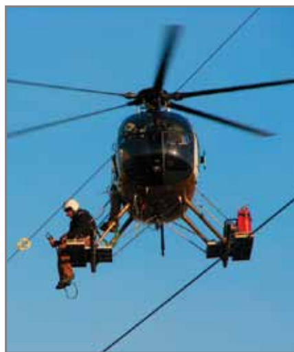
This line worker is attaching bird flight diverters to the wires to reduce the likelihood of birds flying into the wires. Photo courtesy of CapX2020
