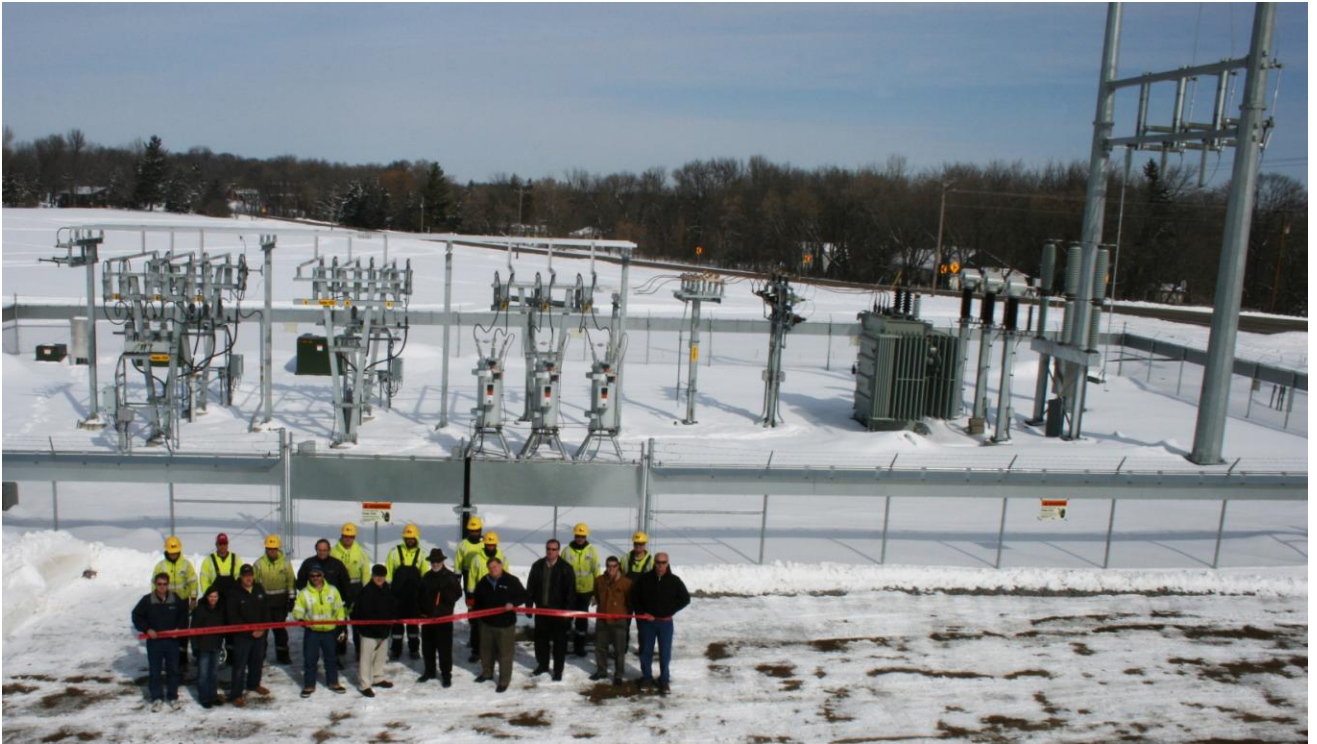
The new Lake Caroline Substation.
