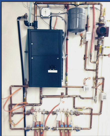
Traditional boiler installation Labor-intensive science project
