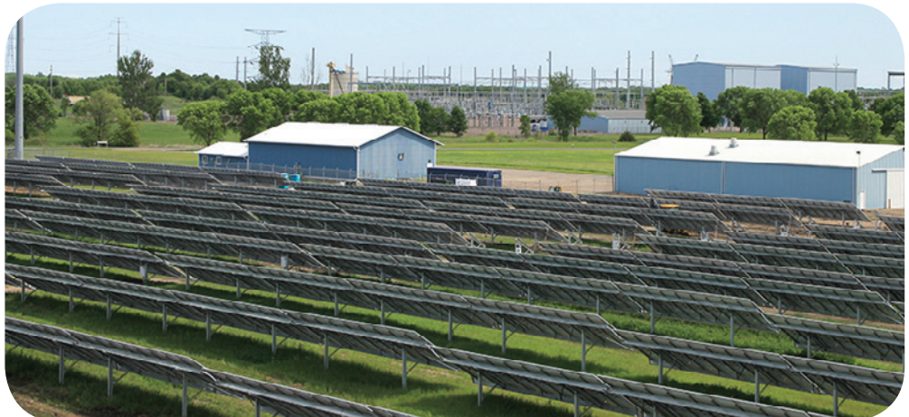
Nearly all of the 8,360 solar panels are mounted at the Dickinson Solar site in Buffalo. The panels will provide approximately 2.25 megawatts of energy to Wright-Hennepin.
